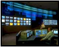
Boston Central Artery/Tunnel
