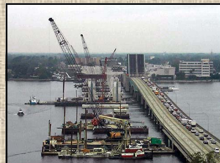
Right: Fuller Warren Bridge, Jacksonville, Florida
